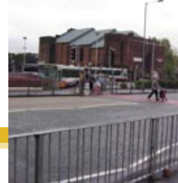
Former cinema building
